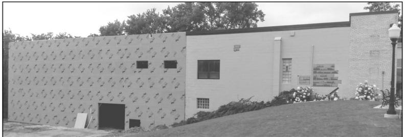
With the framing and sheathing completed for the museum addition, horizontal siding will next be installed to integrate new and old.
