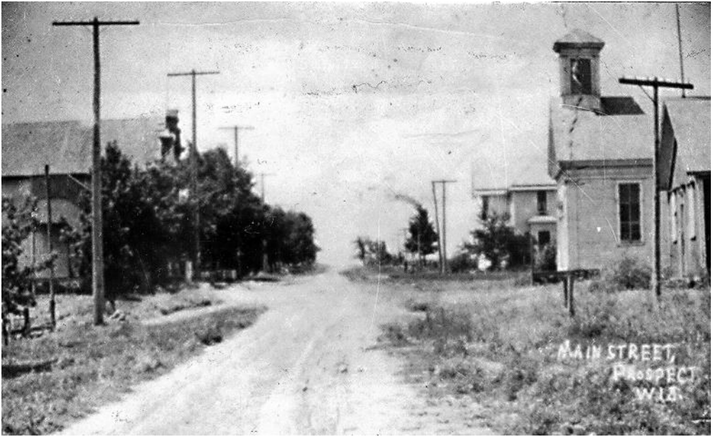
Fig. 5. The traveler passing through the Prospect Hill community ca. 1908 would have this view looking west along National Ave (once known as the road to Mukwonago and here called Main St.). At right are the Prospect school and Freewill Baptist Church. At left is the Winton store.
